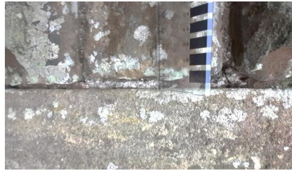
Showing a typical joint with original lime mortar
