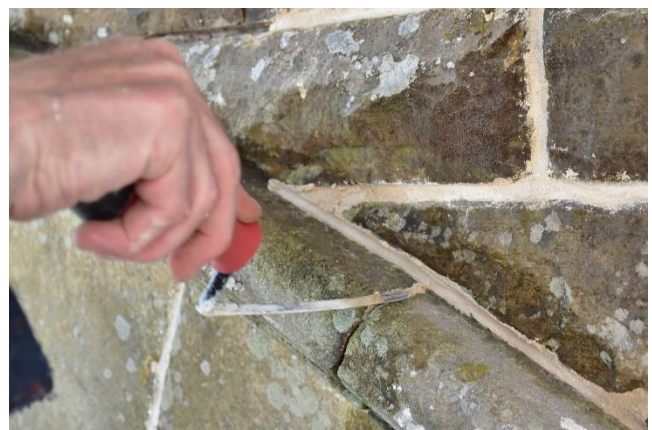
Julian remixing the lime mortar and pointing in progress
