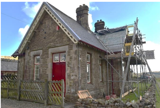
Reinstating the slating (September 2021)
