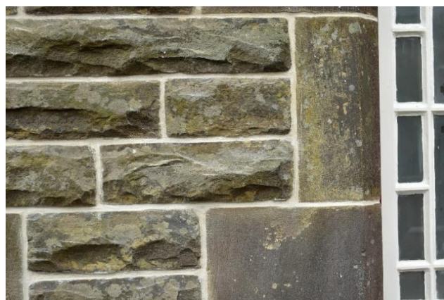
Completed repointing taken on 6 th July 2023
