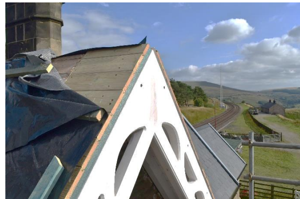
New purlins (showing the bolted connection) and barge board in place (September 2021)
