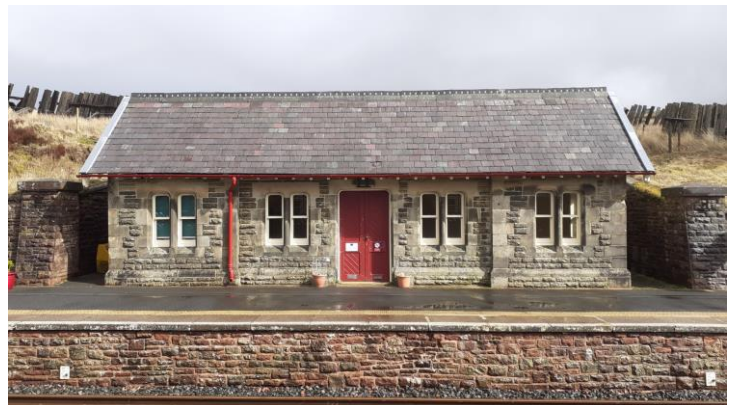
The southbound waiting room following refurbishment.
