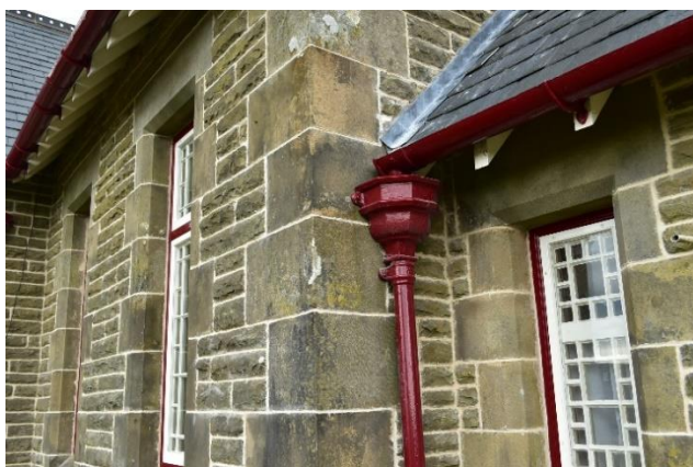
Completed repointing taken on 6 th July 2023
