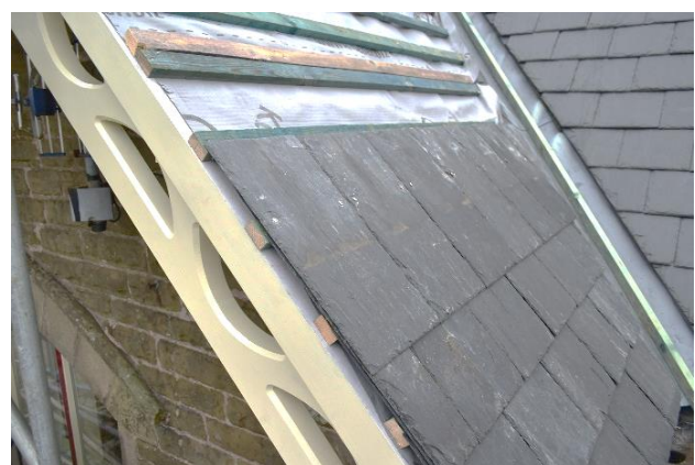
Reinstating the slating (September 2021)
