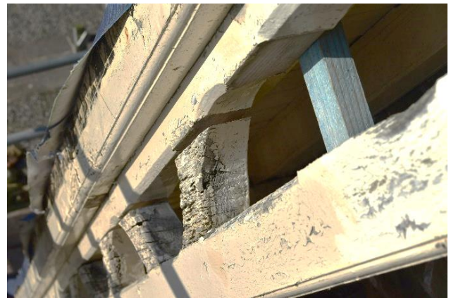
Showing the state of the gable barge boards (2021)
