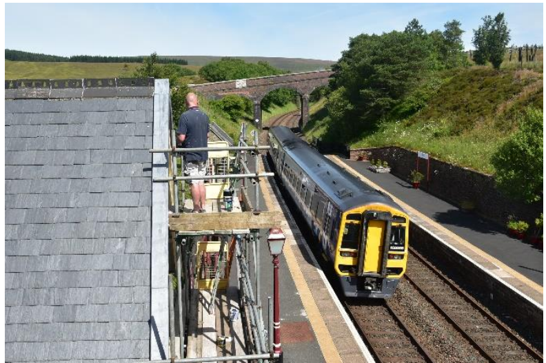
Steven Alderson painting the bargeboard at high level as the mid-afternoon northbound passes on 11 th July 2022
