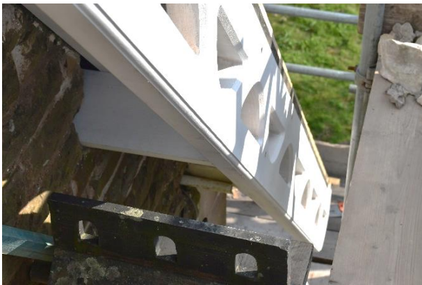
New purlins (showing the bolted connection) and barge board in place (September 2021)
