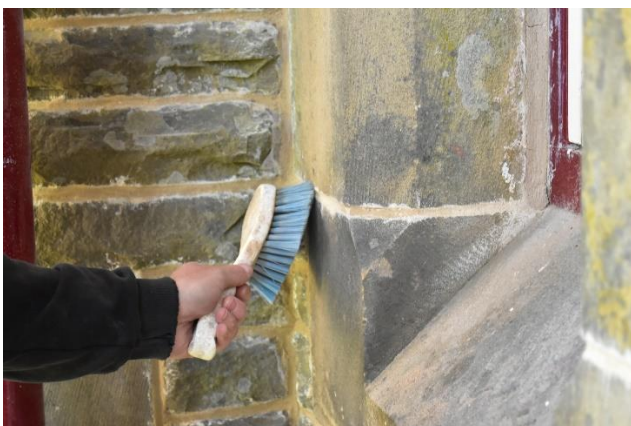
Julian remixing the lime mortar and pointing in progress
