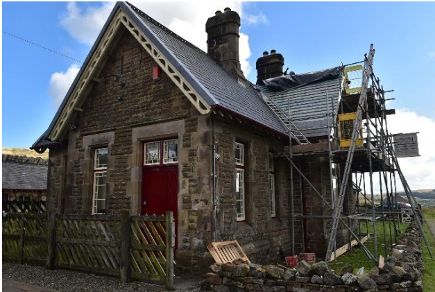
Reinstating the slating (September 2021)
