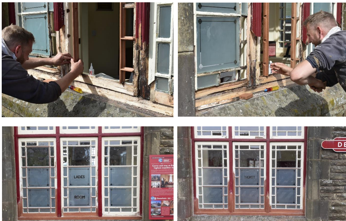
Philip Middleton carefully re-assembling the decayed elements of the windows and the completed work before decoration (June 2022)
