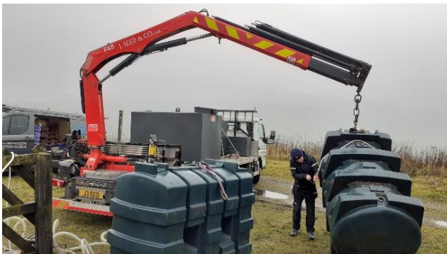
The old fuel tank is removed and the new tank placed into the cattle dock (October 2021)
