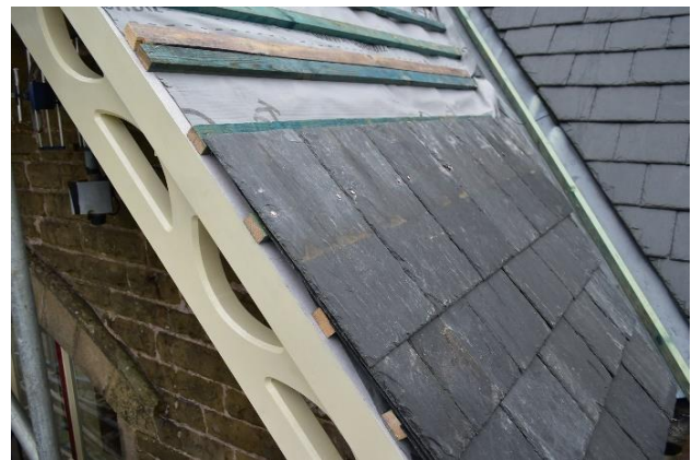
Reinstating the slating (September 2021)
