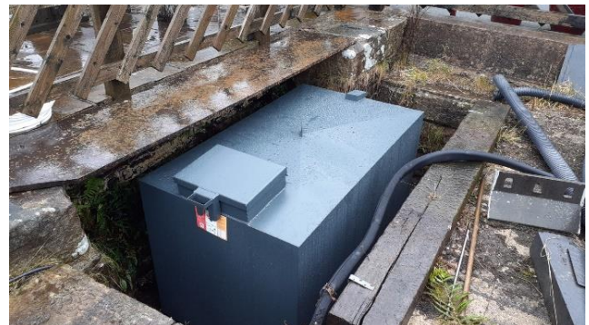
The old fuel tank is removed and the new tank placed into the cattle dock (October 2021)
