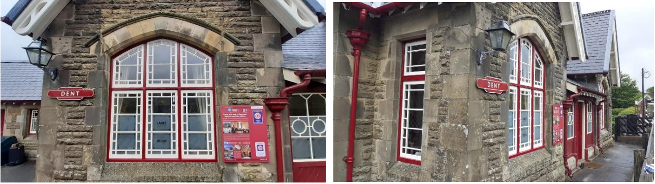
The windows after being painted by Steven Alderson (July 2022)
