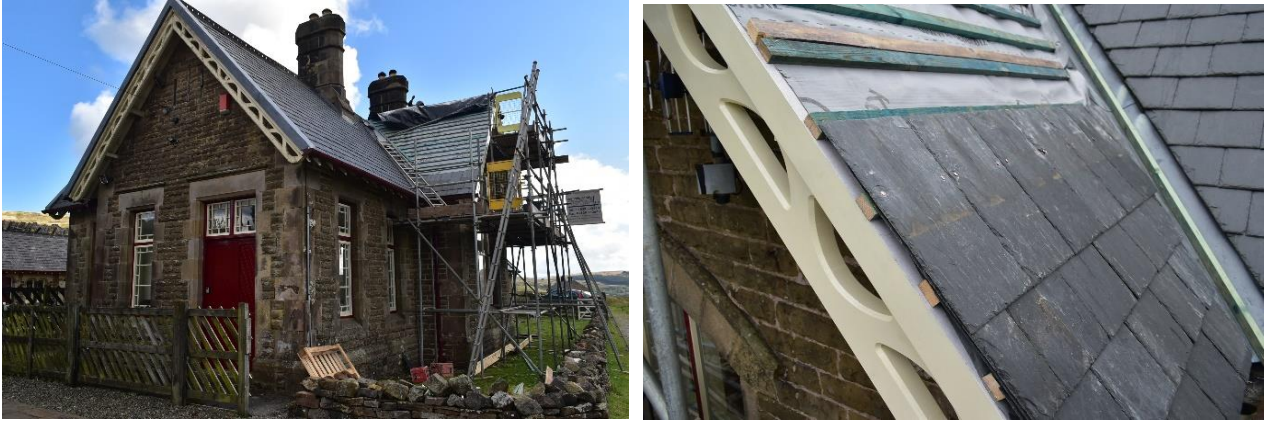
Reinstating the slating (September 2021)
