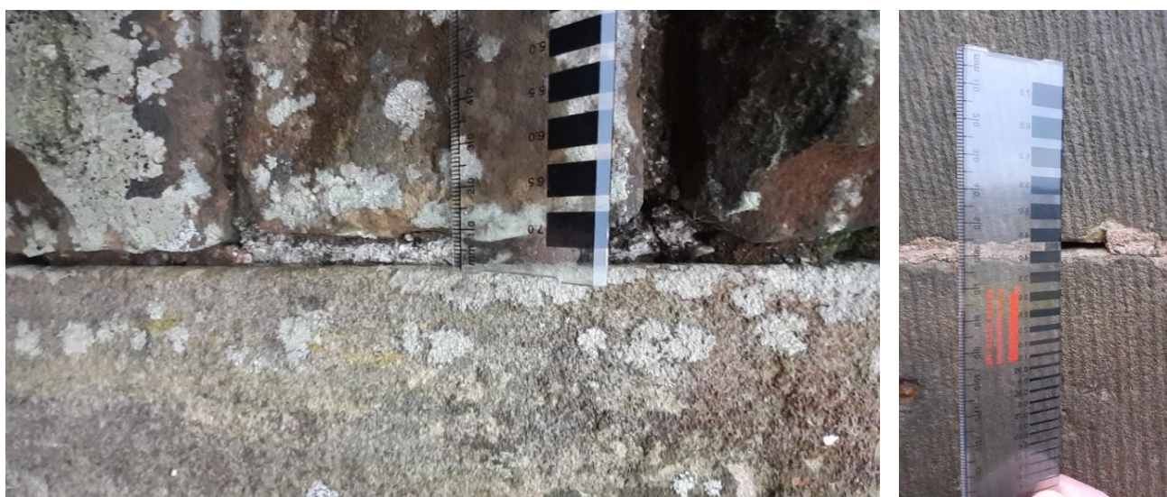
Showing the state of some of the joints and cement patching
