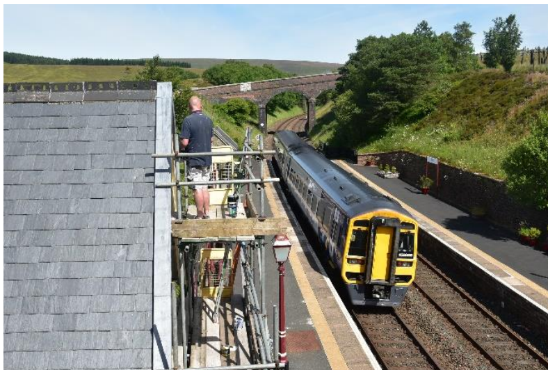
Steven Alderson painting the bargeboard at high level as the mid-afternoon northbound passes on 11 th July 2022
