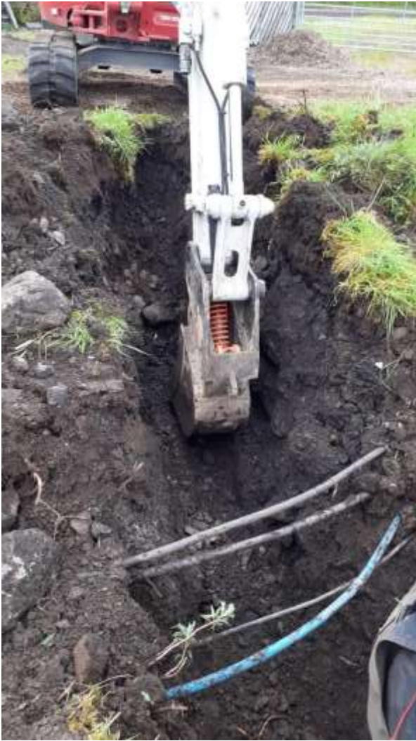
Locating existing service cables and pipes
