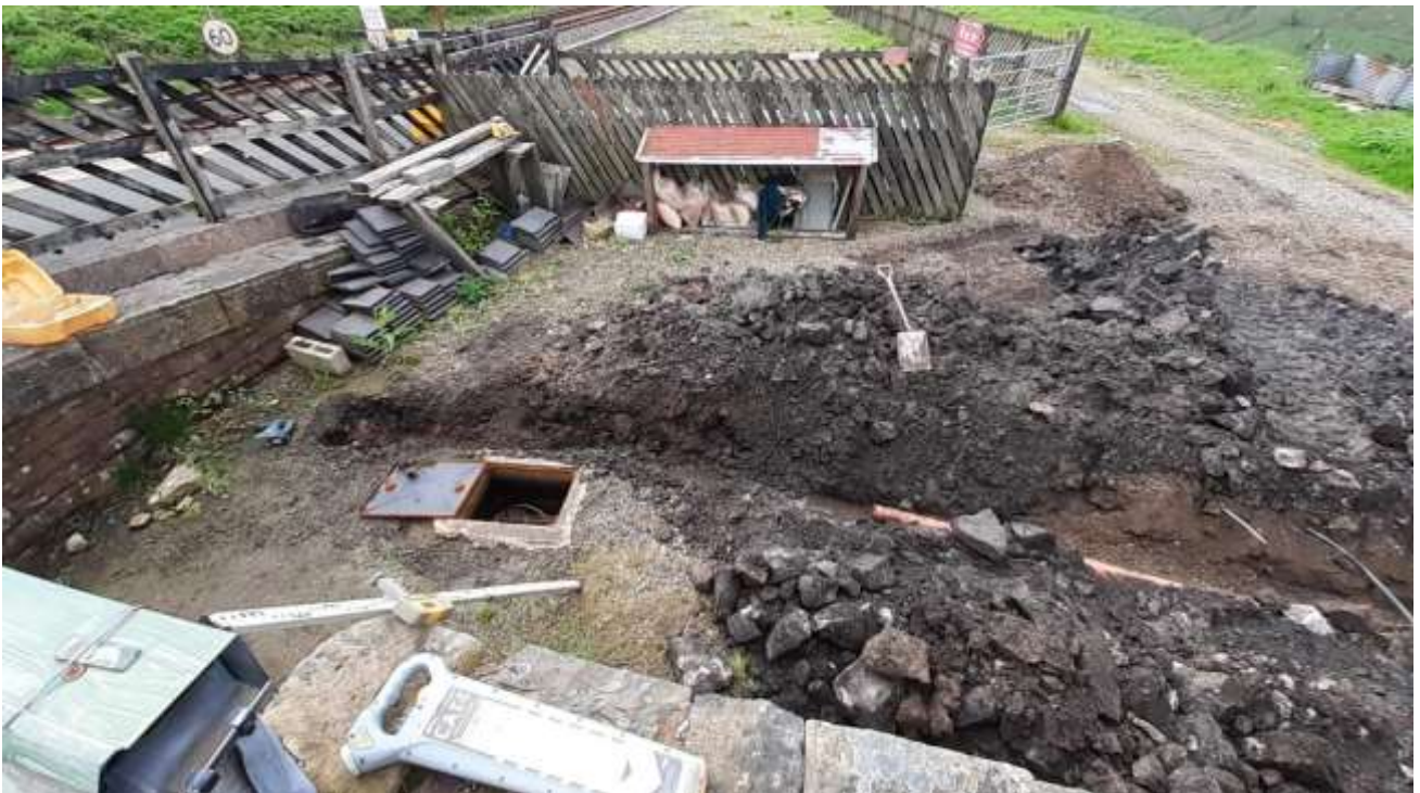
Locating existing service cables and pipes
