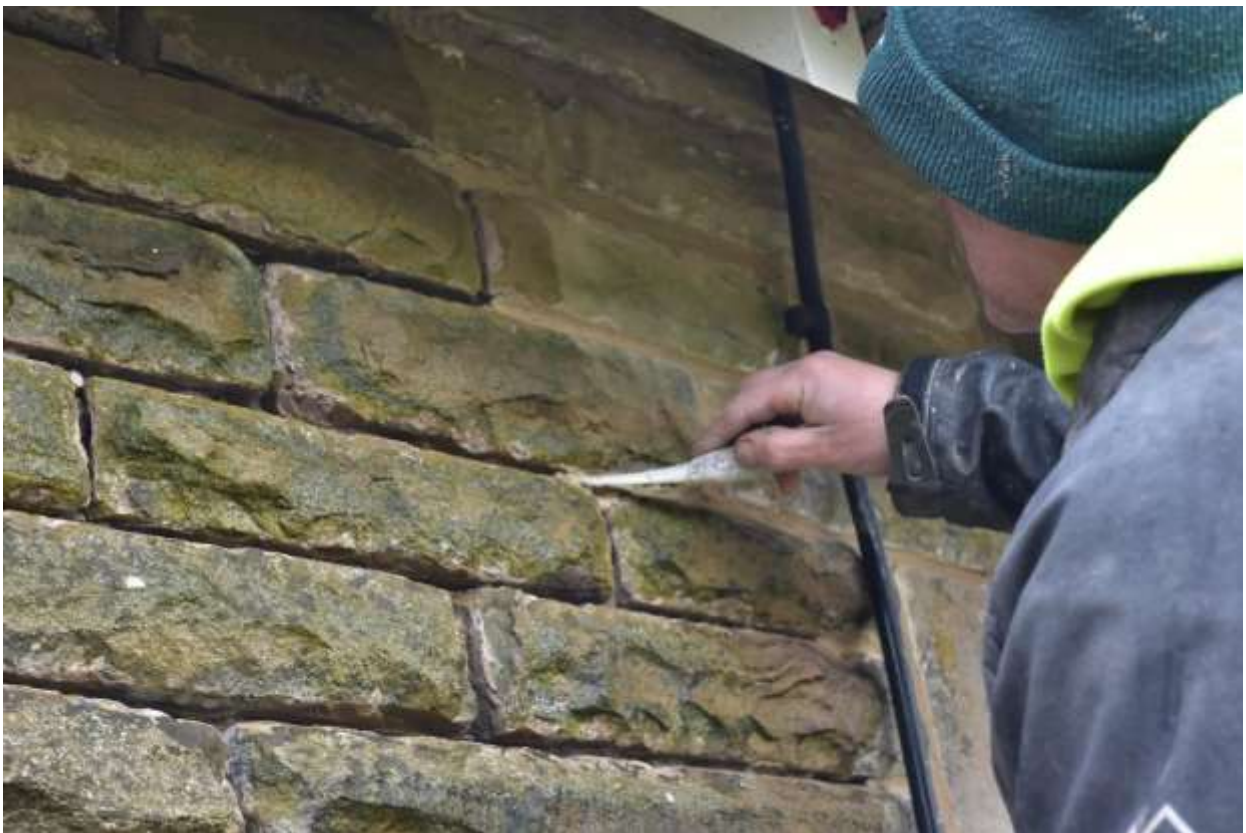
Lime mortar in progress
