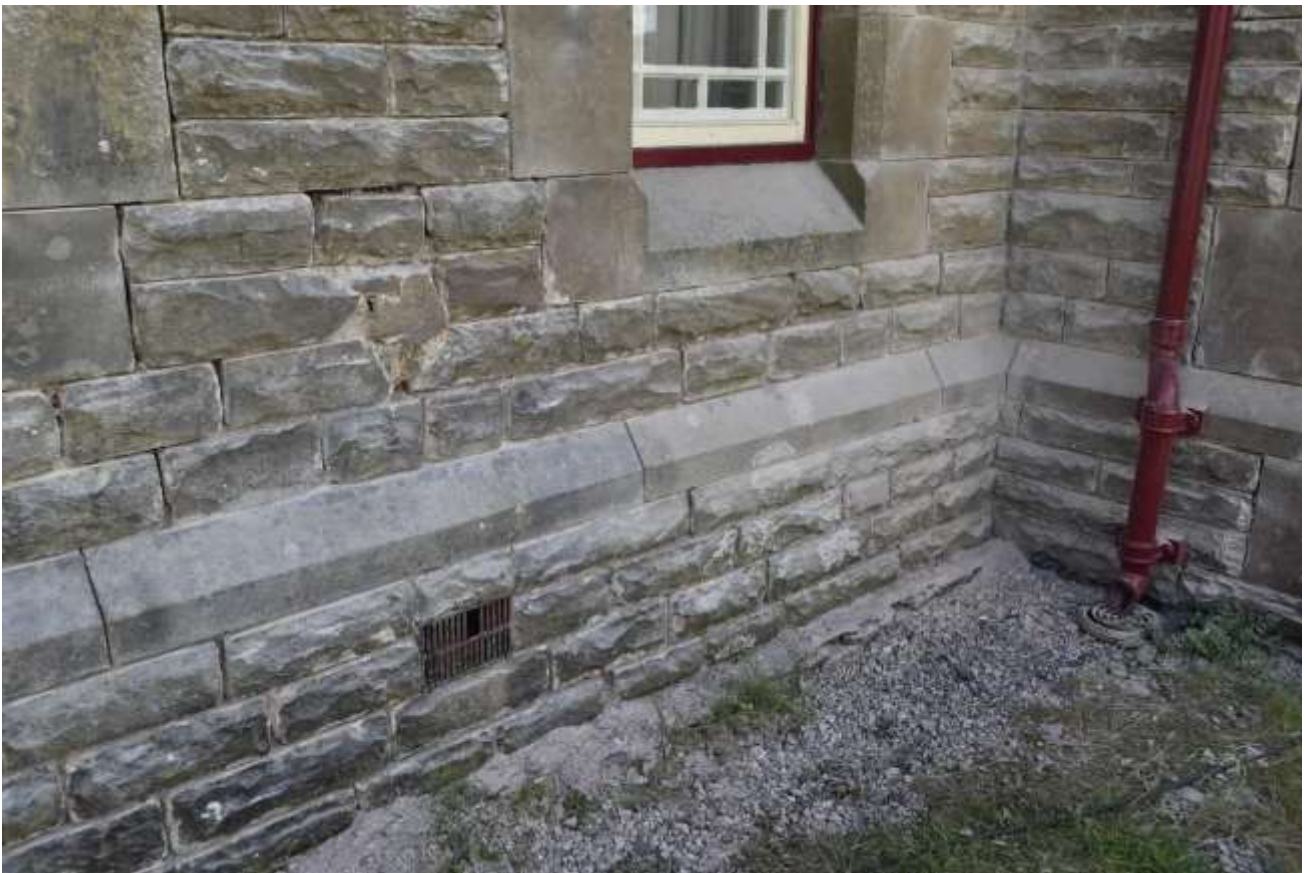
Joints raked out in preparation for pointing
