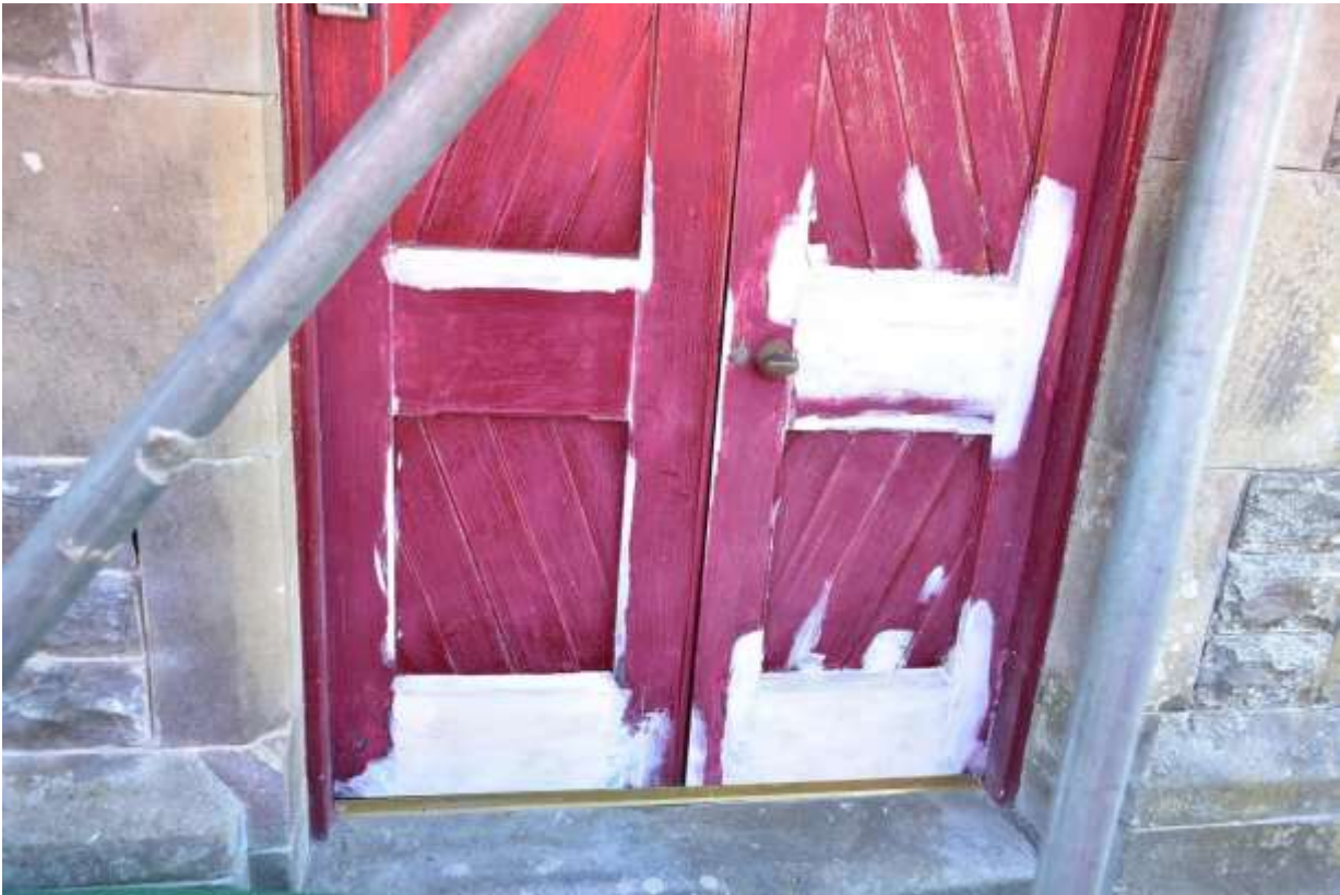
Porter's Room external doors refurbished and primed ready for undercoat.
