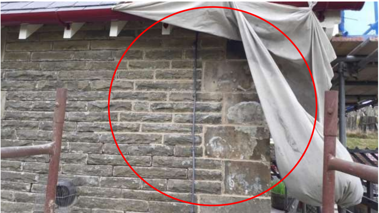
Completed section of mortar
